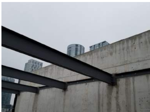
FIGURE 1: Simple beam connection (steel beam to embedded plate) – slotted angle.
