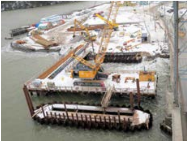
FIGURE 16: Deep foundations using H-Piles
