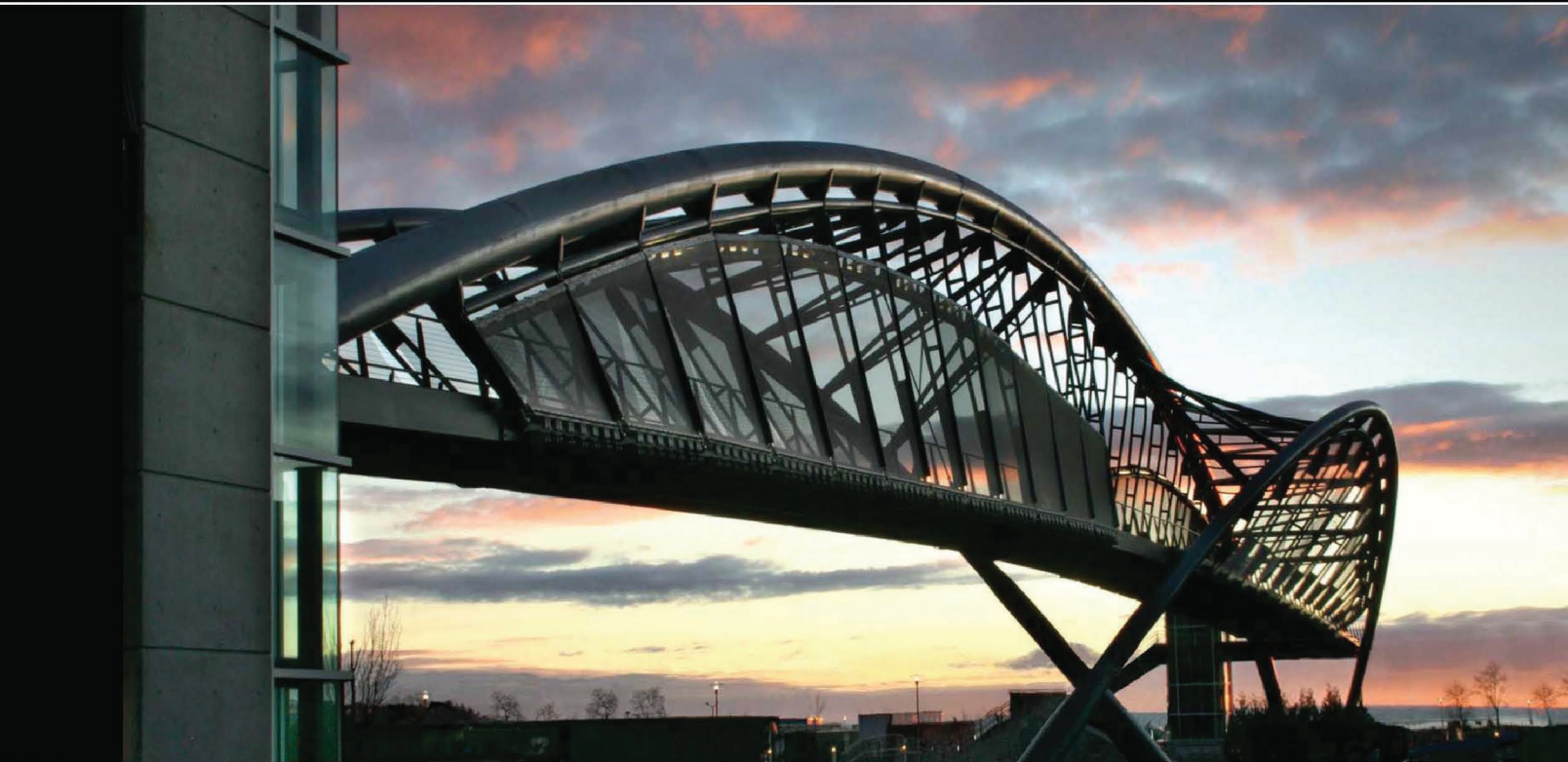
Helix Bridge, Seattle Washington - 36" O.D. x 1.25" wall and 24" O.D. x 1" wall bent to a multiple radius helix
