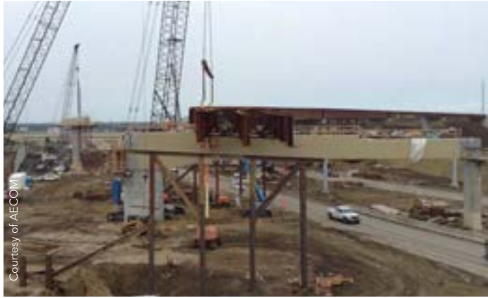
FIGURE 4: Bridge 23.3 Girder Erection (Pier 5 to Abutment 1)
