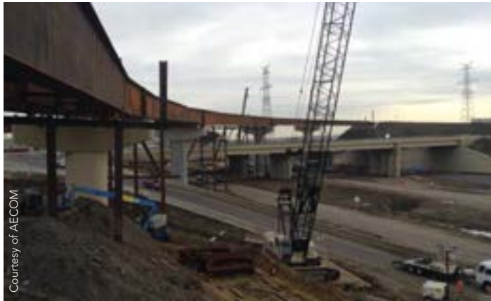
FIGURE 6: Bridge 23.5 Girder Erection Completed (Pier 4 – Abutment 1)
