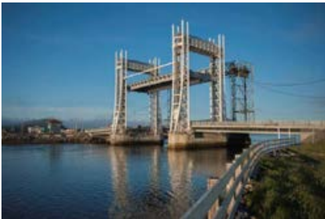
FIGURE 18: Sir Ambrose Shea Vertical Bridge on opening day September 23, 2016
