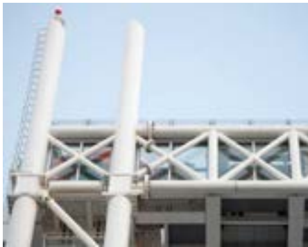
FIGURE 13: Aerial tower view
