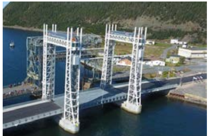
FIGURE 19: Sir Ambrose Shea Vertical Bridge on opening day September 23, 2016
