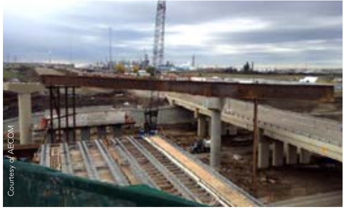
FIGURE 5: Bridge 23.5 Girder Erection (Pier 1 to Pier 2)
