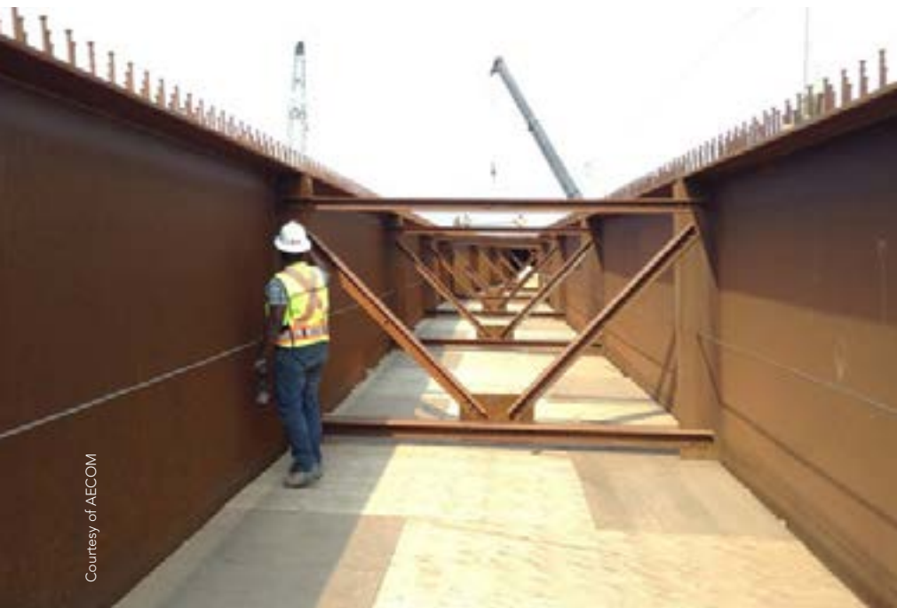
FIGURE 3: Bridge 23.3 Girder Cross Frames
