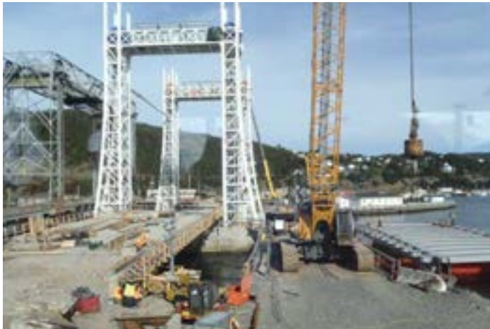
FIGURES 5 & 6: Erection using a crane from a temporary work trestle
