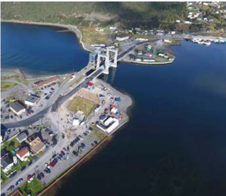
FIGURE 2: Both the new and existing lift bridges cross the Placentia Gut
