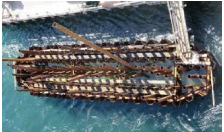
FIGURE 17: Pipe piles at pier foundation
