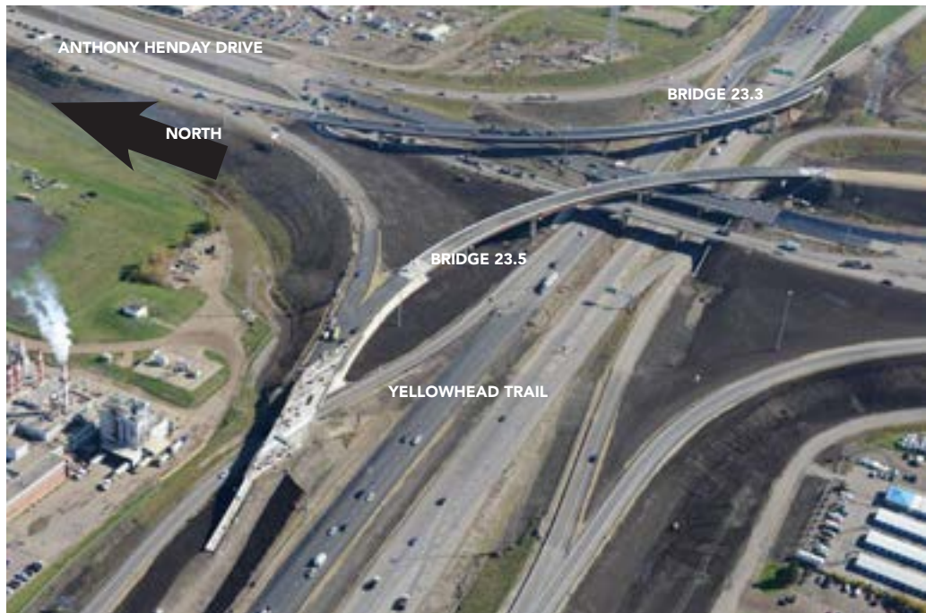
FIGURE 1: Anthony Henday Drive / Yellowhead Trail Interchange near completion
