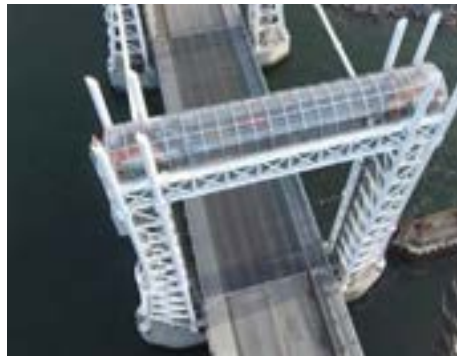
FIGURE 14: Aerial tower view
