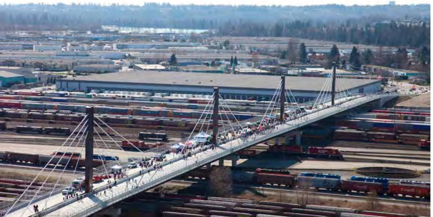
The Coast Meridian Overpass in Vancouver is an excellent example of a cable-stayed bridge
