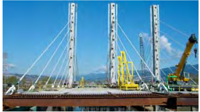
Construction on the Pitt River Bridge
