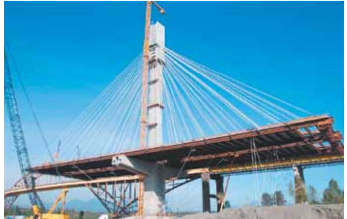
The $1.9-billion Port Mann Bridge project in Vancouver
