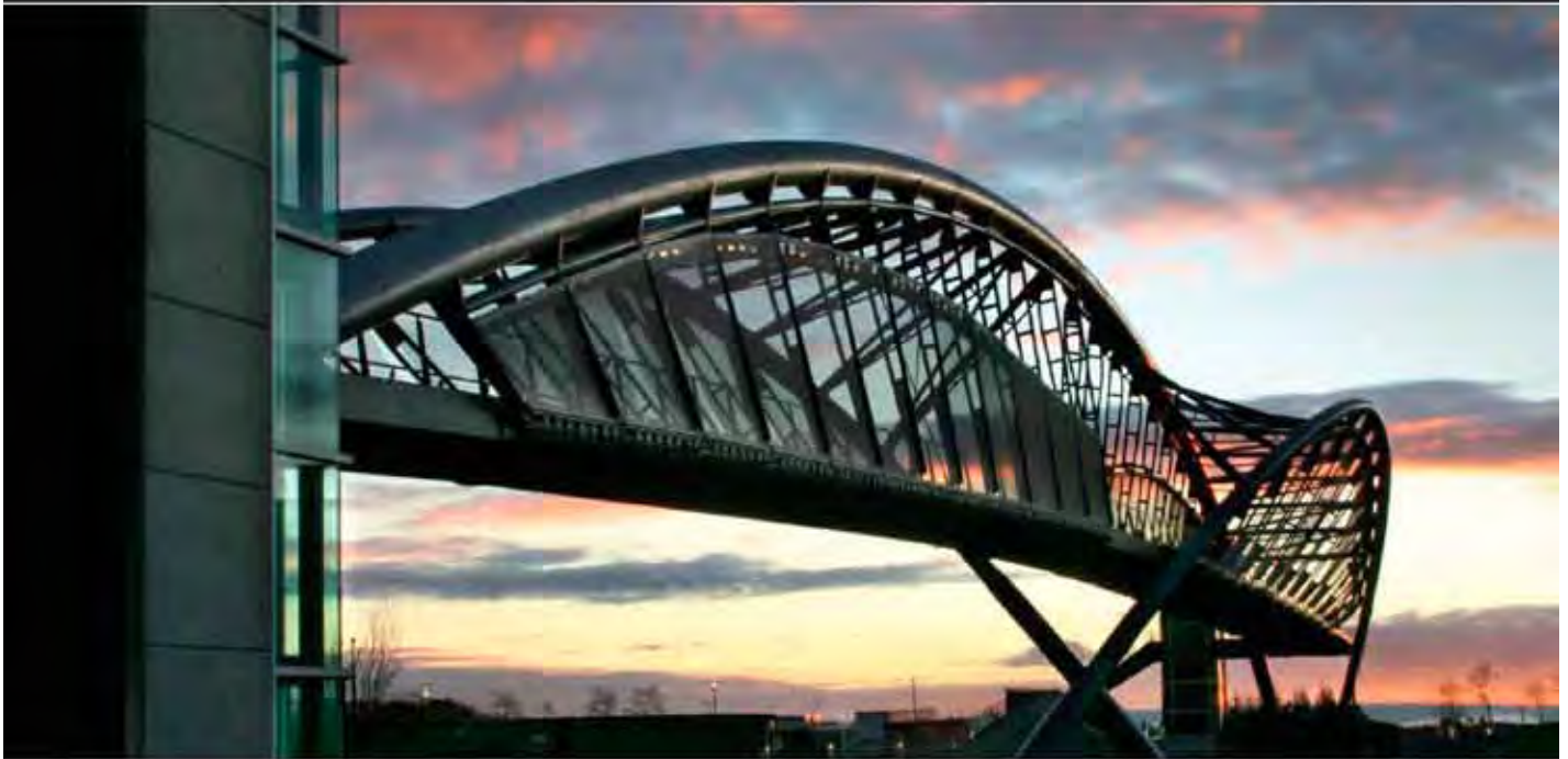
Helix Bridge, Seattle Washington - 36" O.D. x 1.25" wall and 24" O.D. x 1" wall bent to a multiple radius helix
