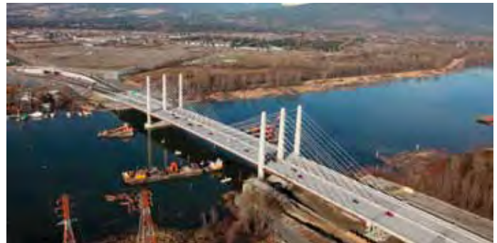
The Pitt River Bridge completed
