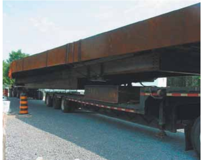
Picture showing the transportation rig with the special stiffening frame
