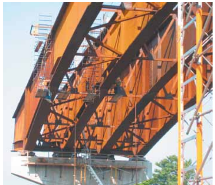
Haunched pier segments over the piers
