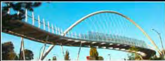
Griffiths Drive Pedestrian Bridge, Burnaby, BC - 24" O.D. x 7/8" wall
