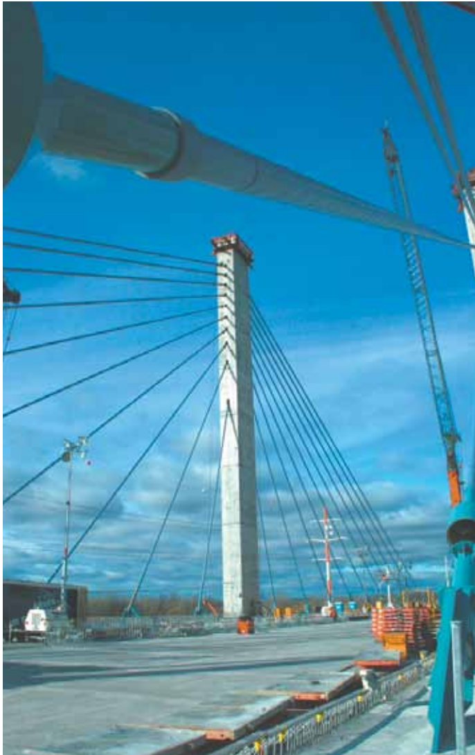
The bridge comprises an innovative steel framing system
