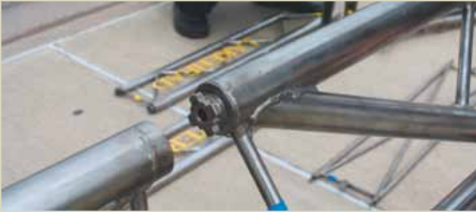
The "camera connection" developed by the Lakehead University steel bridge team was both very efficient in transferring load and quick to assemble
