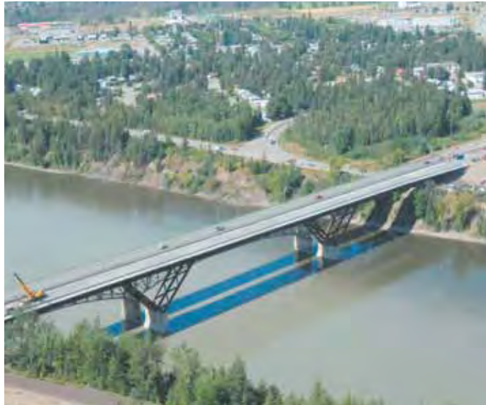
The Simon Fraser Bridge supports a concrete deck with two traffic lanes
