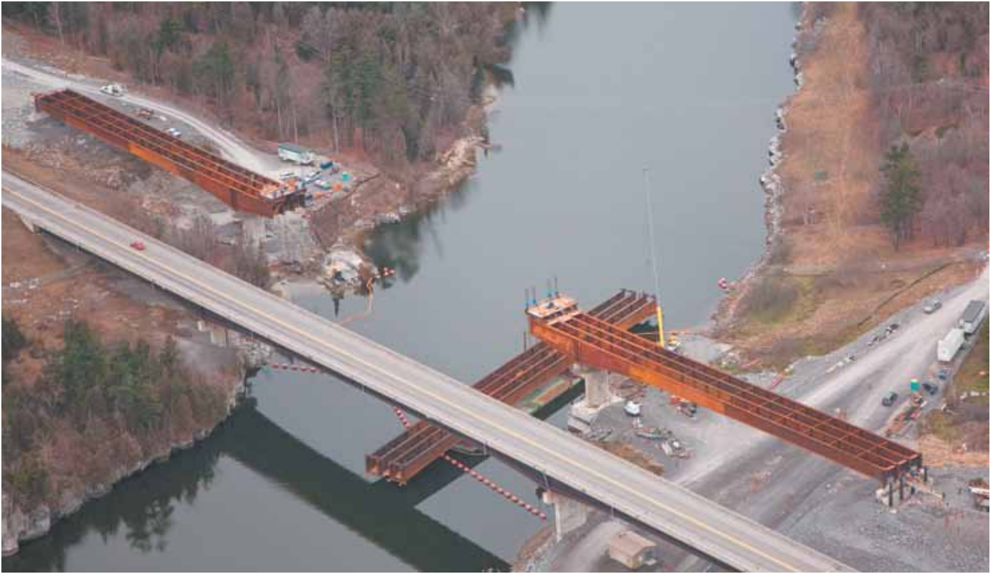
Assembly of the central span segments on the barge completed
