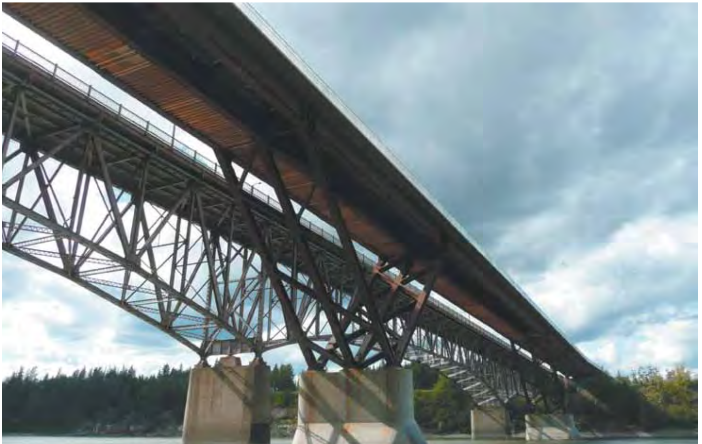
The new Simon Fraser Bridge has a total length of 400 metres
