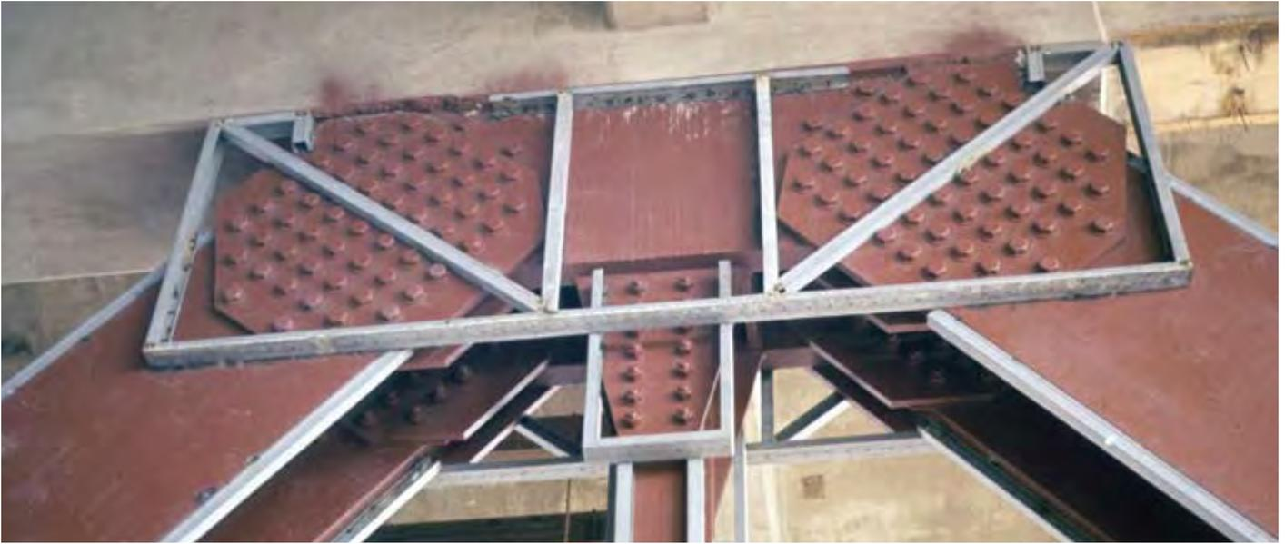
Protected steel truss – thermal barrier with gypsum board (before application with furring channels attached)
