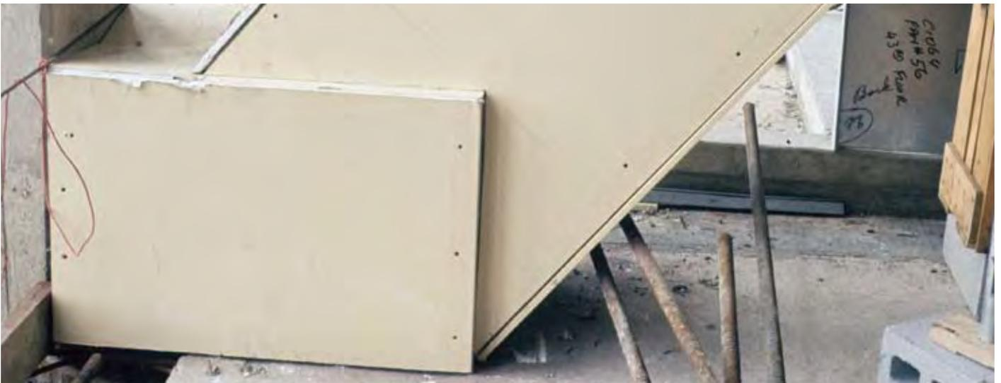
Protected steel truss – thermal barrier with gypsum board
