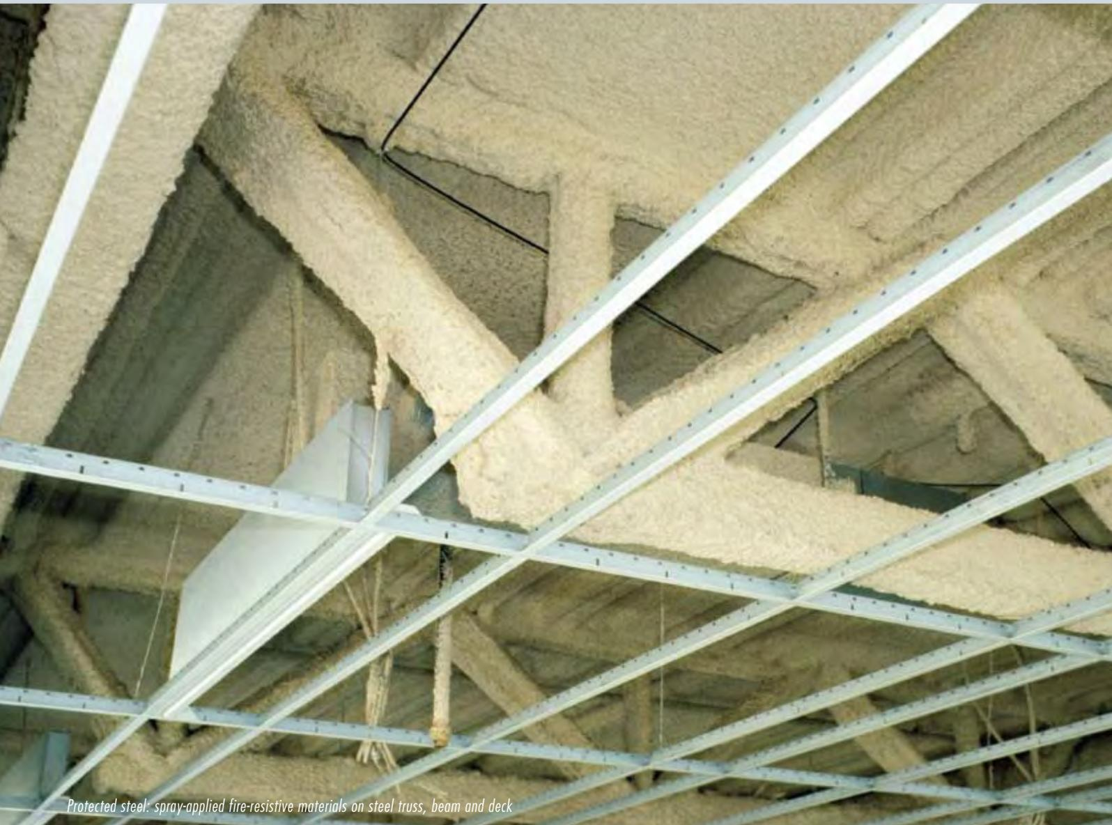
*Protected steel: spray-applied fire-resistant materials on steel truss, beam and deck*
