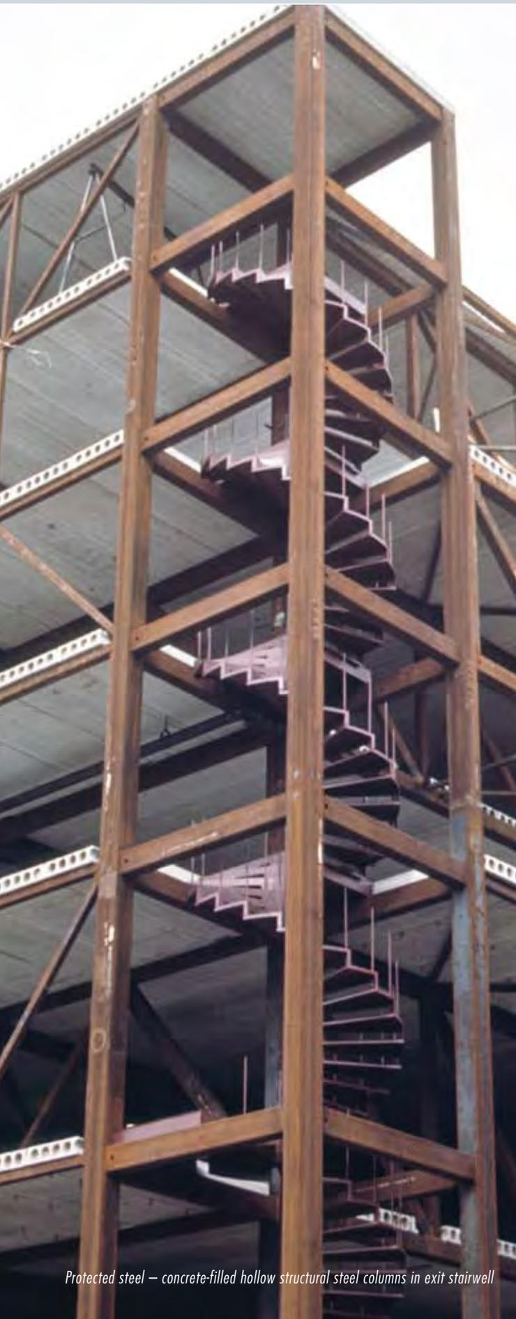
Protected steel – concrete-filled hollow structural steel columns in exit stairwell
