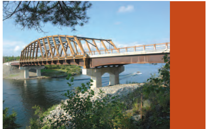
PROJECTS CONVERTED TO STEEL AWARD Award of Merit Replacement of Sioux Narrows Bridge
