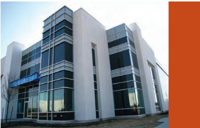
Award of Merit Orlando Speculative Industrial Warehouse
