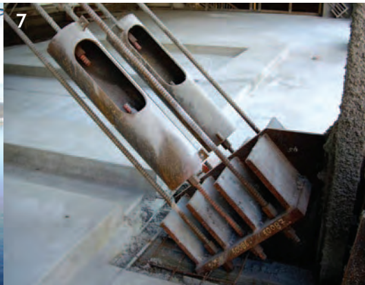
(6) "Outside – in" architecture embraced the views of the City, Stanley Park, Burrard Inlet and North Shore mountains with clear glass perimeter walls soaking in the view. (7/8) High capacity springs were created from cupped spring washers to provide a mechanism to resist lateral loads produced by leaning column, yet allow the building to sway under seismic loading without interrupting seismic energy dissipation. The system also functions as a seismic centering mechanism.
