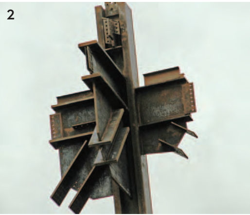
(1) SAP Model for 3D analysis was translated directly to other programs for structural modeling. (2) Complicated steel joints made simple(r) with the use of Tekla detailing software. The Tekla model was built in the Structural Engineering office and was provided to the fabricators as a 3D design model for their use.
