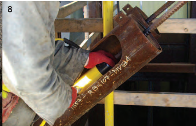
(6) "Outside – in" architecture embraced the views of the City, Stanley Park, Burrard Inlet and North Shore mountains with clear glass perimeter walls soaking in the view. (7/8) High capacity springs were created from cupped spring washers to provide a mechanism to resist lateral loads produced by leaning column, yet allow the building to sway under seismic loading without interrupting seismic energy dissipation. The system also functions as a seismic centering mechanism.
