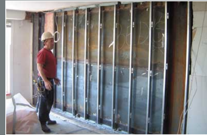
3) Replace the metal studs and the insulation.
