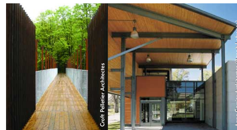
Steel as the primary structural system and wood as the secondary system (sheathing, decking)
