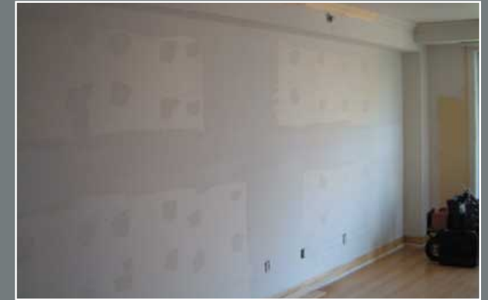
4) And close with gypsum panels!
