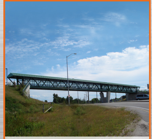
North Bay Pedestrian Bridge, Ontario
