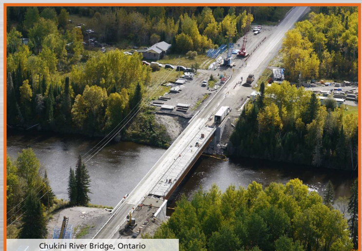
Chukini River Bridge, Ontario
