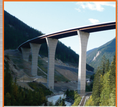
Kicking Horse Canyon - Park Bridge, British Columbia
