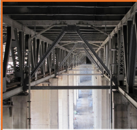
Hogg's Hollow Bridge, Ontario
