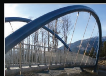
Stawamus Pedestrian Bridge, Sea-to-Sky Hwy 99, BC - 20" O.D. x 3/8" wall
