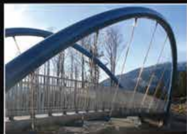
Passerelle Stawamus, Sea-to-Sky Hwy 99, C.-B. – 20 po (DE) x 3/8 po (paroi)
