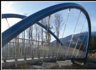
Passerelle Stawamus, Sea-to-Sky Hwy 99, C.-B. – 20 po (O.D.) x 3/8 po (paroi)
