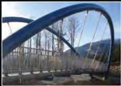
Passerelle Stawamus, Sea-to-Sky Hwy 99, C.-B. – 20 po (O.D.) x 3/8 po (paroi)
