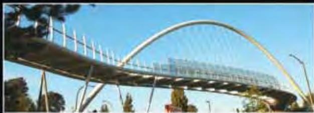
Passerelle Griffiths Drive, Burnaby, C.-B. – 24 po (O.D.) x 7/8 po (paroi)
