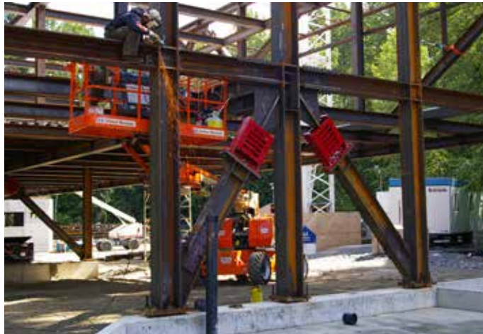
Audain Art Museum: Design by Patkau Architects; Fabrication by George Third & Son; Cast Connex Scorpion Yielding Connectors
