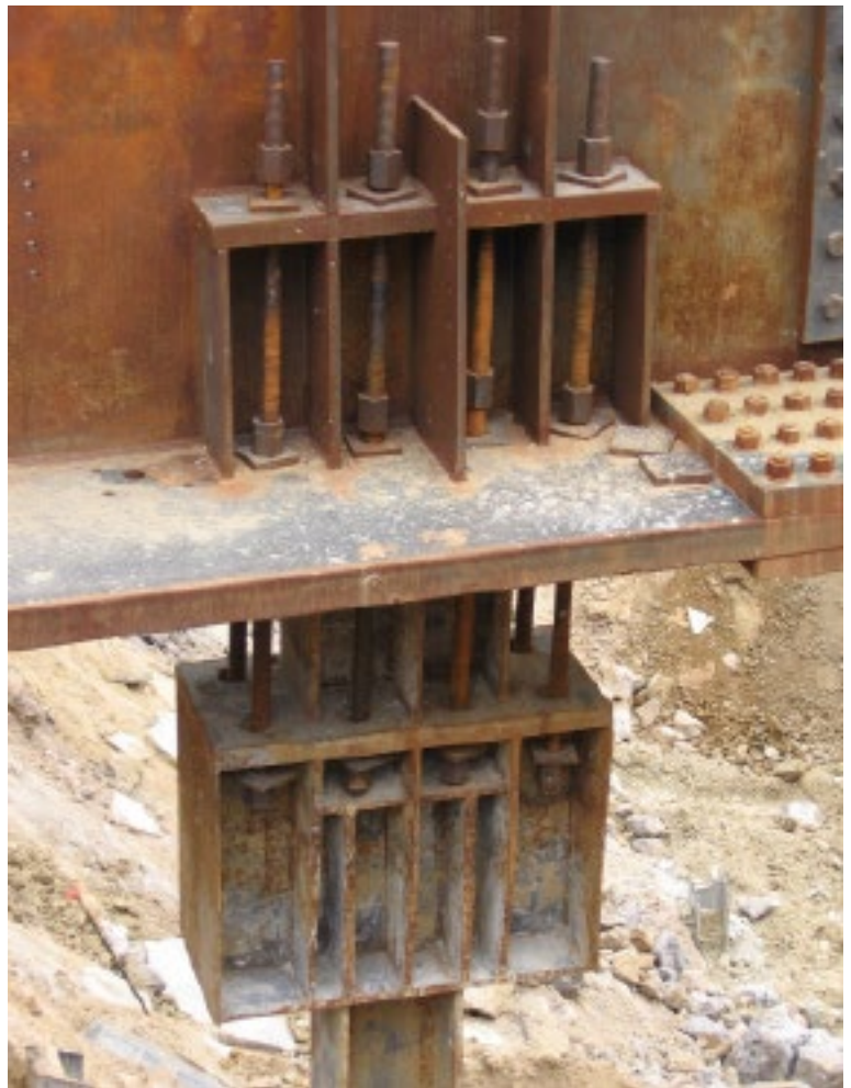
EIGHT HYDRAULIC JACKS WERE INSTALLED ON THE EXTERIOR GIRDERS TO ELIMINATE THEIR INITIAL CAMBER
