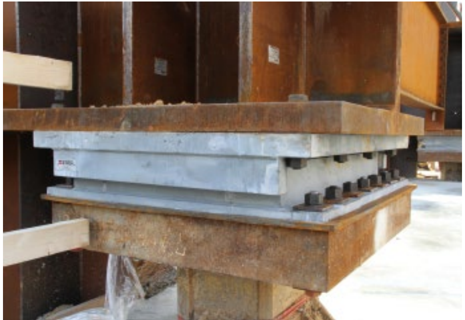
ONE END OF EACH GIRDER RESTS ON A SLIDING BEARING TO TRANSFER MOVEMENTS CAUSED BY TEMPERATURE VARIATIONS
