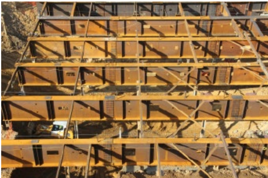
EIGHT MAIN GIRDERS SUPPORT THE 15 CONCRETE-FRAMED UPPER FLOORS
