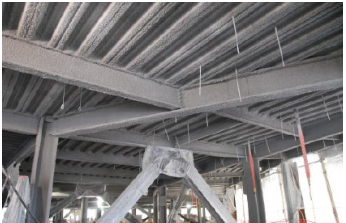
PROTECTED STEEL - SPRAY-APPLIED FIRE- RESISTIVE MATERIALS ON STEEL BEAMS AND STEEL DECK
