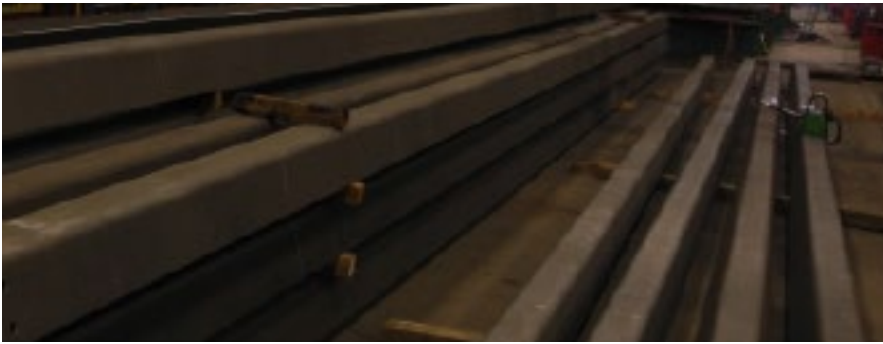
FIGURE 2: LONGITUDINAL RIBS BEFORE THEIR ASSEMBLY ON THE DECK PLATE
