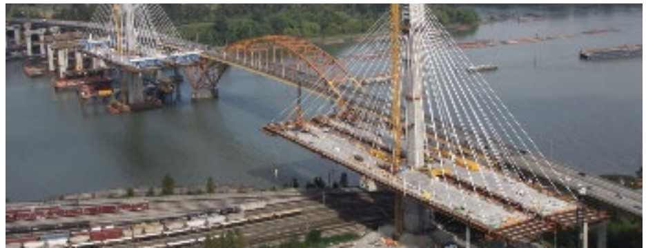
FIGURE 6: GENERAL ERECTION LAYOUT
