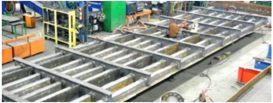
FIGURE 3: WELDING OF THE TRANSVERSE COMPONENTS OF AN ORTHOTROPIC PANEL
