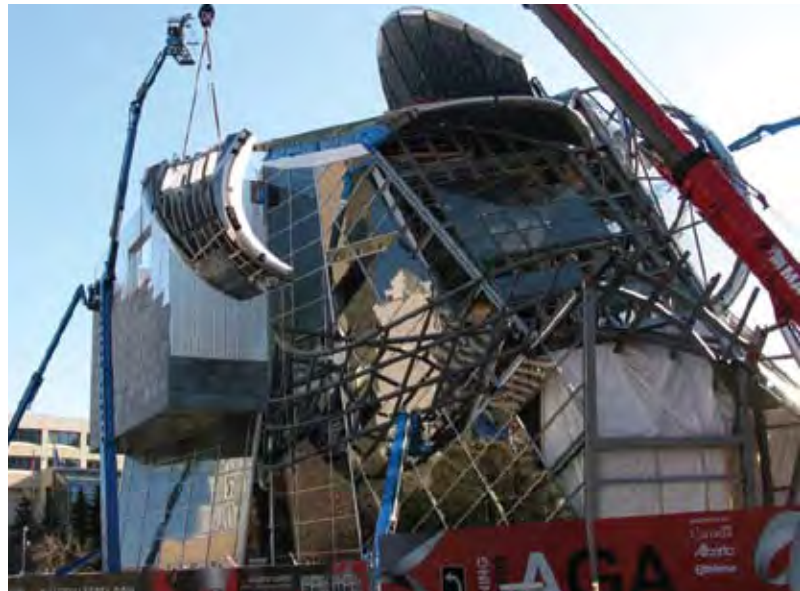
Erection of a pre-clad section of borealis frame
