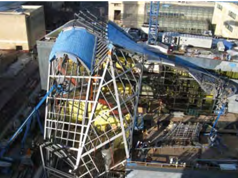
Atrium and roof framing: borealis frame on the terrace roof being “skinned”
