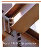
ANSWER: Knife edge angle connection, commonly known as knife connection, is a very common type of beam shear connection. It features a pair of angles that are typically welded to the column in the shop and bolted to the beam web in the field (Figure 1). While knife connection serves as a popular beam shear connection, its use is not
