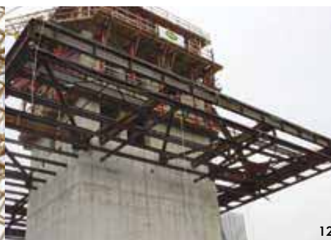
The erection of the two-storey steel trusses required a complicated connection between the steel trusses and the concrete core, involving massive steel plates, embedded in the concrete. This interconnection required close co-ordination between the steel fabricator, the rebar contractor and the formwork contractor, as well as with the general contractor.
