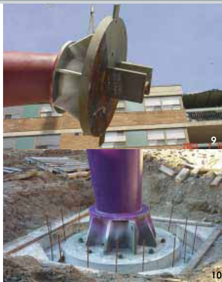
A key connection on the OCAD building was between the steel columns and the caissons supporting them. There was little margin for error to set the anchor rods.
