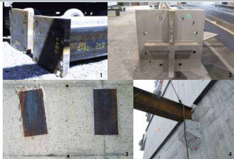
Load transfer from one material to another - Base plates that only need to transfer compression typically have 4 anchor rods (1). When lateral forces are important, shear keys can be used (2). Situations not shown include large plates that need to resist important overturning moments, or systems that need to transfer important forces in tension. Embedded plates provide load transfer from steel beams to the concrete core (3) but need to be properly positioned during the concrete pour! Another alternative for connecting to the core is a seat, either in concrete (4) or steel.
