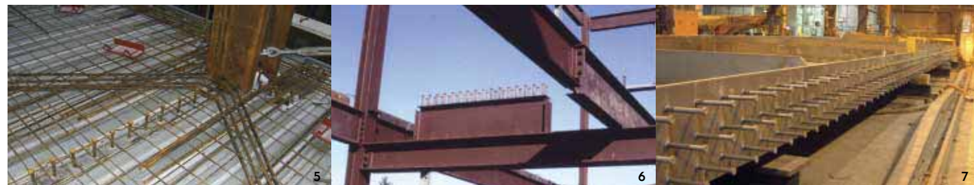
Composite action / floors - Shear studs are used to provide composite action. Studs are welded to the top flange or chord (5) and covered completely with concrete. A composite floor which is ideal in combination with a concrete core is the stub-girder system (6), which acts as a Vierendeel truss, spanning anywhere from 8-12 metres. Today, all steel bridges are composite (7).
