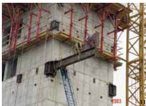
The erection of the two-storey steel trusses required a complicated connection between the steel trusses and the concrete core, involving massive steel plates, embedded in the concrete. This interconnection required close co-ordination between the steel fabricator, the rebar contractor and the formwork contractor, as well as with the general contractor.
