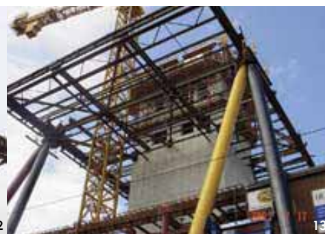
The erection of the two-storey steel trusses required a complicated connection between the steel trusses and the concrete core, involving massive steel plates, embedded in the concrete. This interconnection required close co-ordination between the steel fabricator, the rebar contractor and the formwork contractor, as well as with the general contractor.
