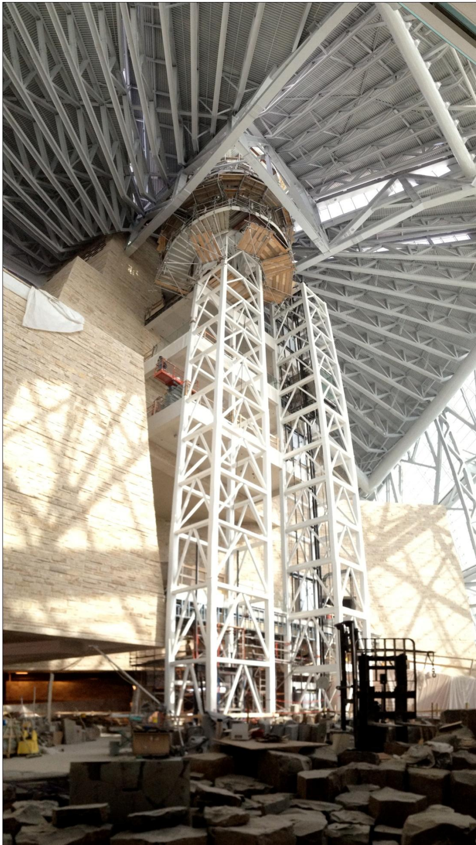
Atrium Elevators and Cloud Roof Antoine Predock Architect PC
