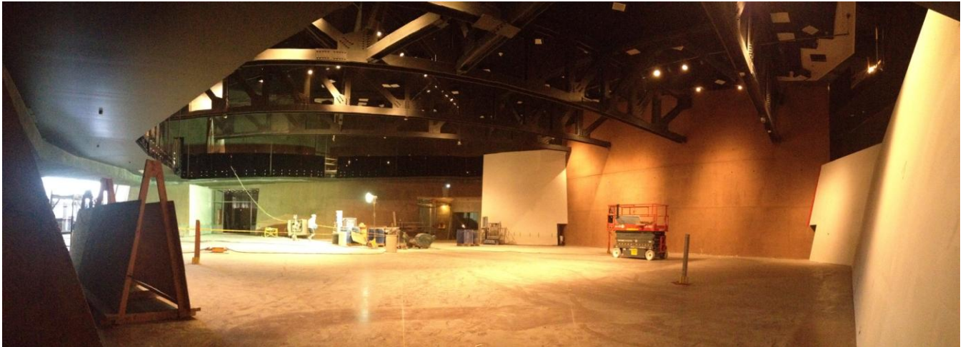
Long Span Trusses below the Garden of Reflection Antoine Predock Architect PC
