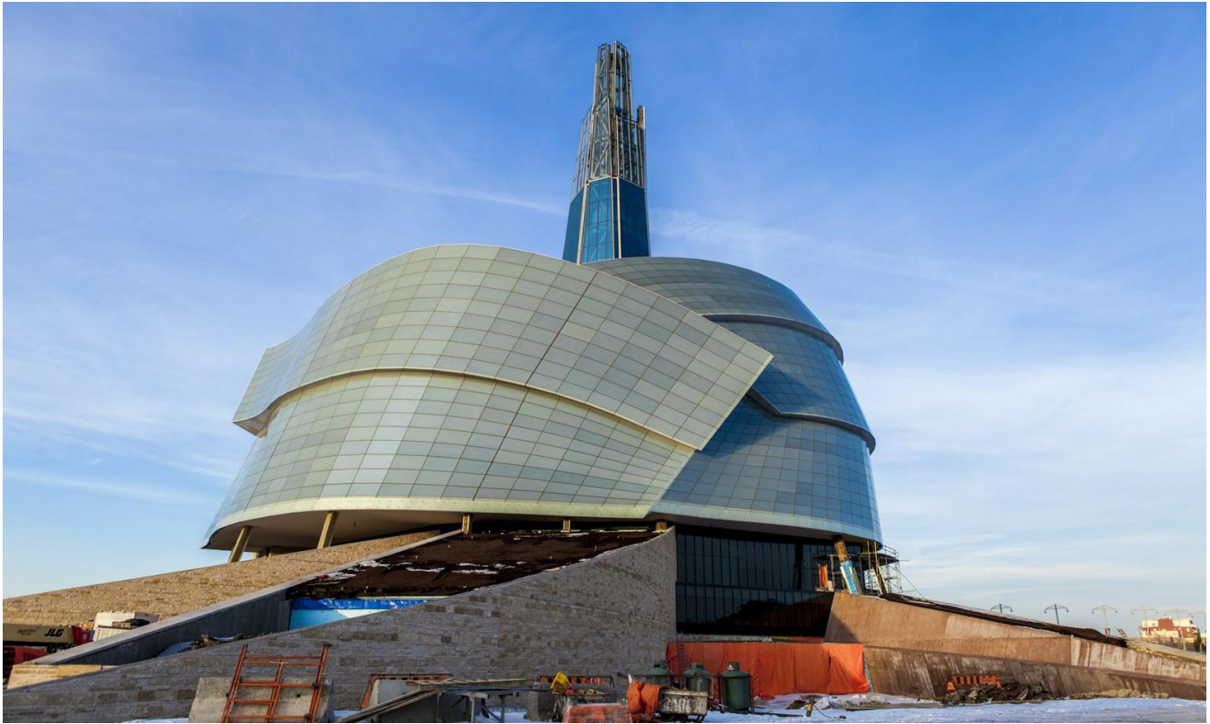
Construction Progress, March 13th 2013 Antoine Predock Architect PC
