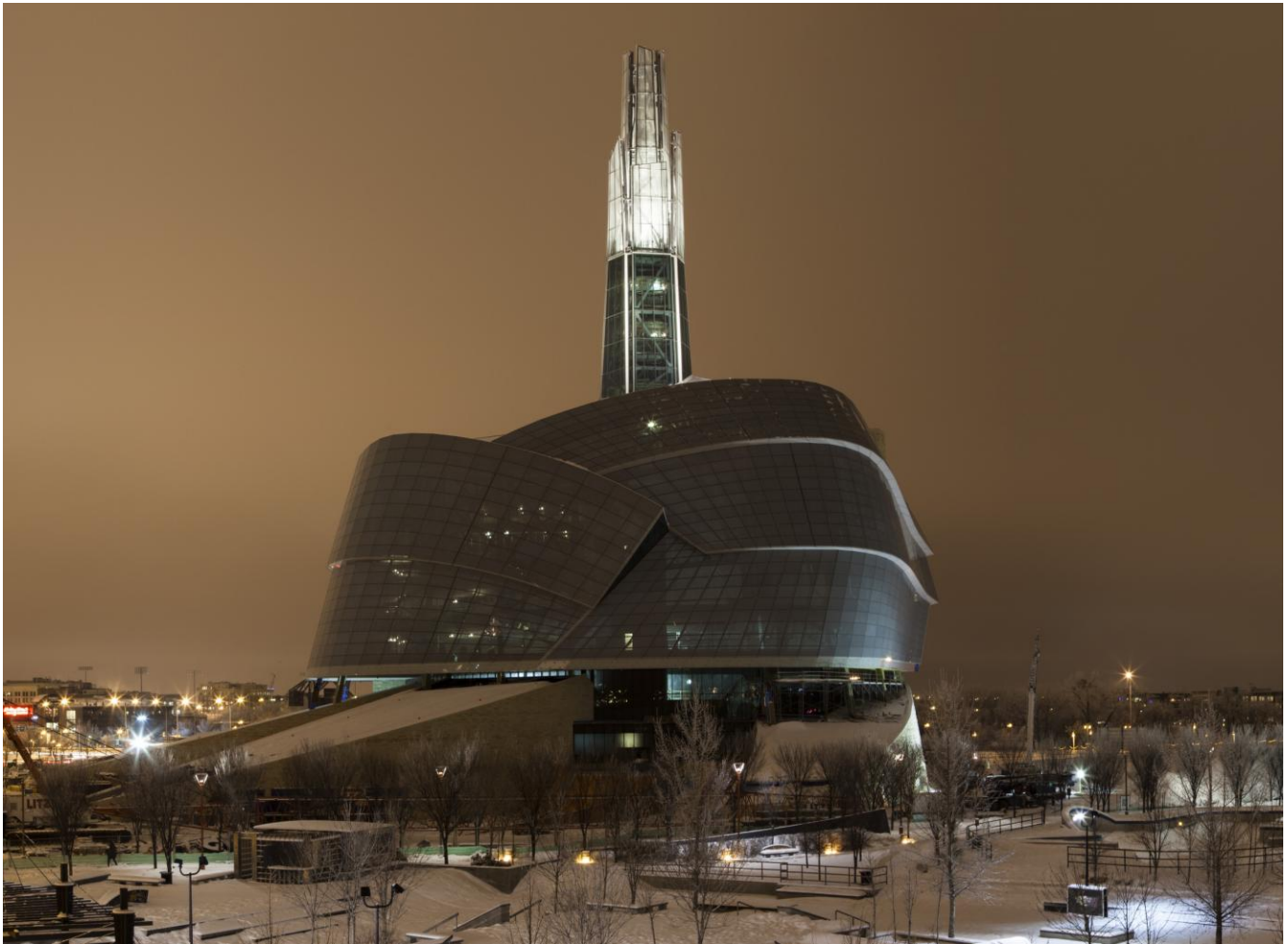
Construction Progress, Winter 2012 Antoine Predock Architect PC
