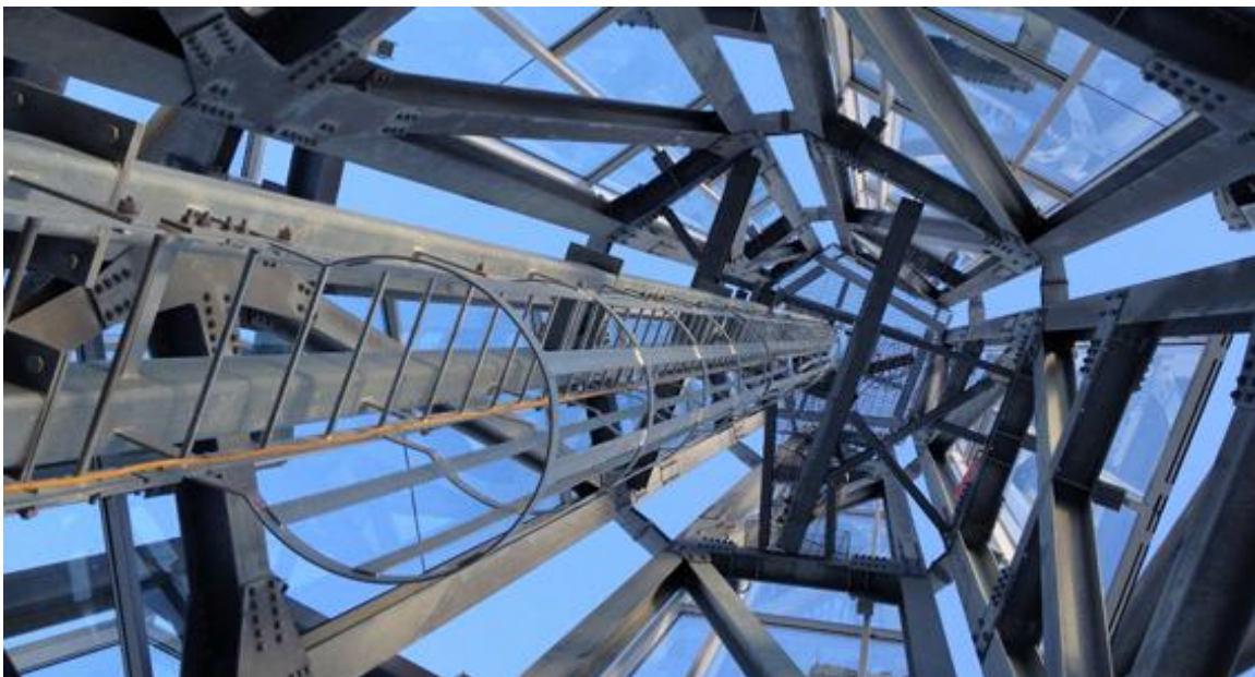
Maintenance Access within the Tower of Hope Antoine Predock Architect PC
