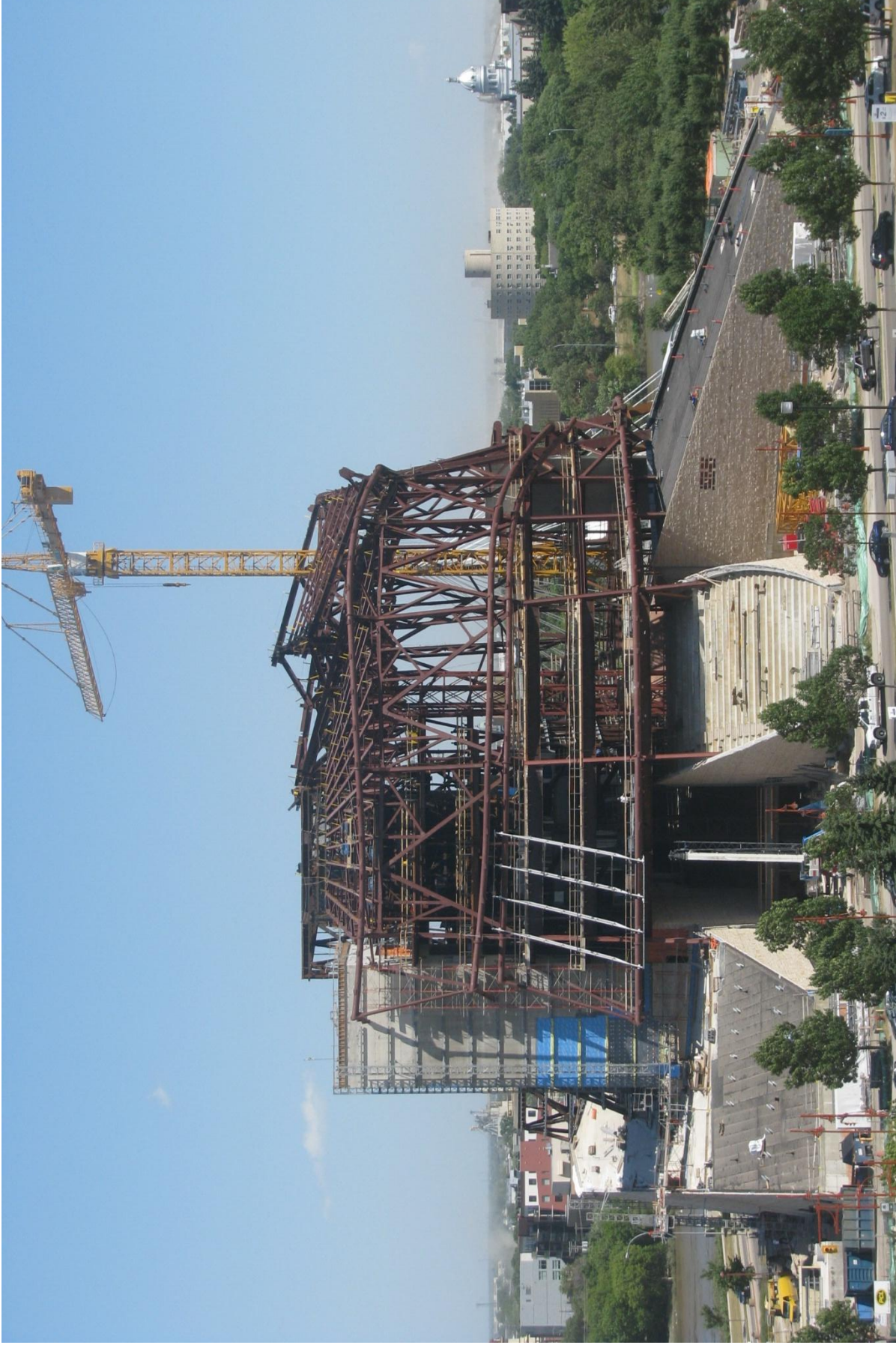
Steel Erection Progress, July 2011
